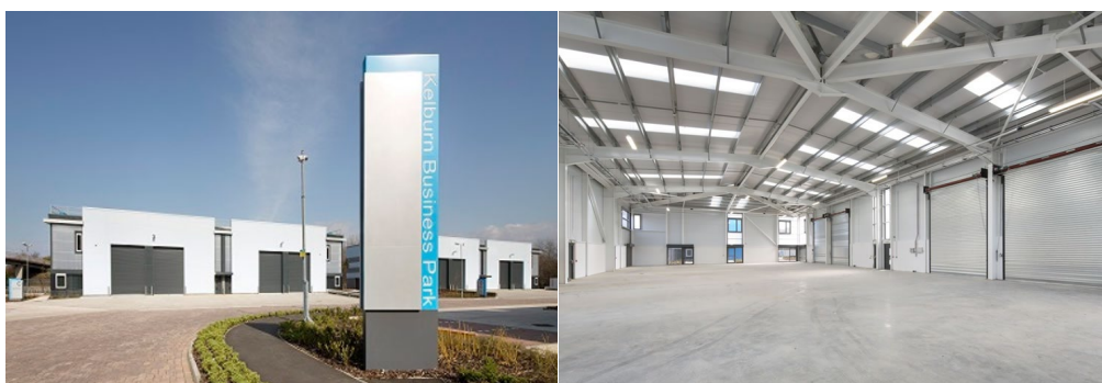
Image 2 Kelburn Business Park Phase 1. Project preparation has commenced for Phase 2.
