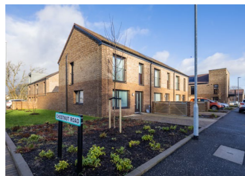
Image 8 New Affordable Housing Development in Inverclyde
